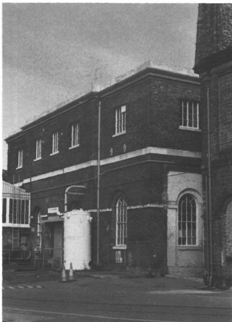
A view of the engine and boiler house designed by John Rennie and later modified by the Navy Board. The boiler, as shown by the original plans, was situated in the central part of the building while the two wings served as engine houses. Designed to accommodate a 50 h.p. Boulton and Watt engine, this was apparently removed in 1929 when it was replaced by electrically-operated machinery.
